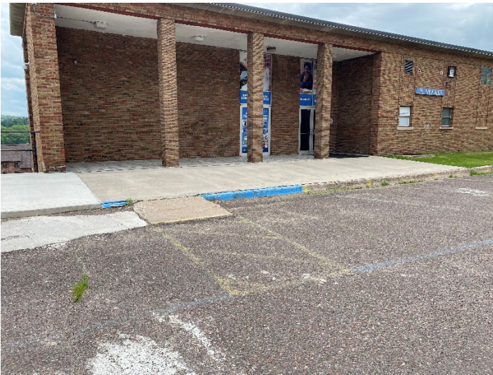
NE Entrance (Summit Street Parking Lot)
