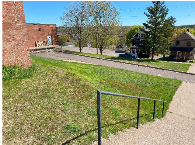
Service Drive on West Side of Building
