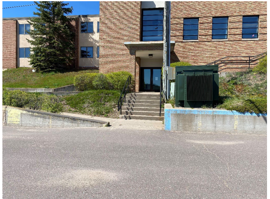
SW Building Entrance (Franklin Street)
