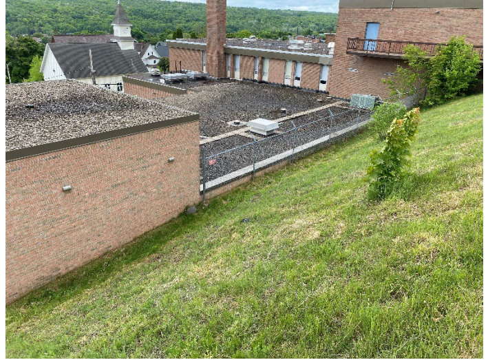
Fence Along Roof
