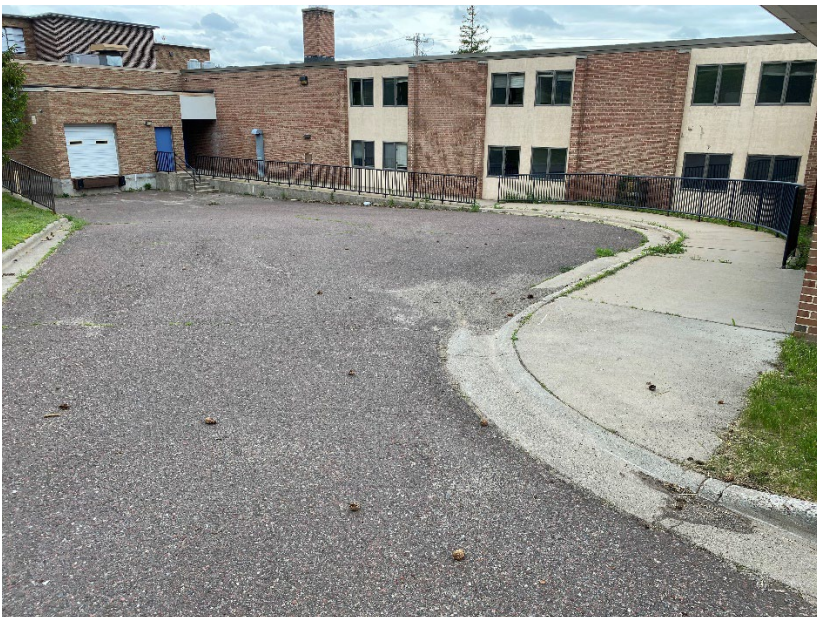
Service Drive to North Side of Building
