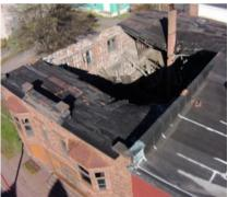
Known as Hermann Flats, this two story sandstone building was built in 1898. Originally a mixed-use space this building was converted to all apartments in 1917. The building is currently very deteriorated; the roof has collapsed leaving behind the sandstone shell. Efforts are underway to stabilize the structure including removal of all structural debris and stabilizing the tops of the walls. The site is served by municipal water and sewer.
