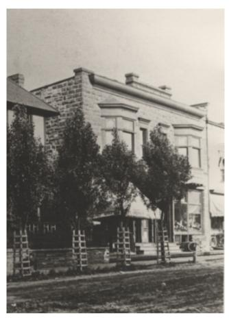
Joseph Hermann had this combination commercial-residential building constructed. The walls of uncoursed ashlar sandstone are complemented by a pressed metal cornice and window hoods. High-grade purer red sandstone is used on the front, while the side and rear are of a poorer grade. The 48' x 68' building had two stores on the first floor; the plate-glass windows have been replaced with brick infill. On the second floor, denoted by two pressed-metal oriels, were two flats, each of nine rooms.
